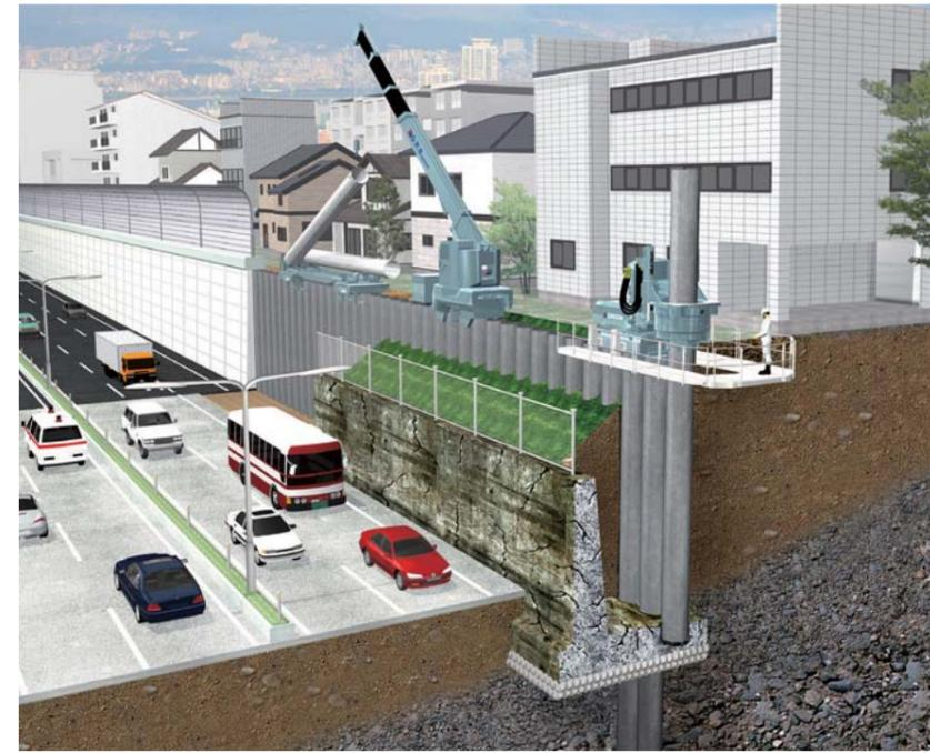
Retaining wall can be easily constructed by continuous tubular pile wall with interlock pieces. Urban function is able to be evolved without disturbing active traffic and surrounding environment even at urban congested area by GRB System that various construction machines such as Clamp Crane, and other associated machines work on the top of tubular piles.
