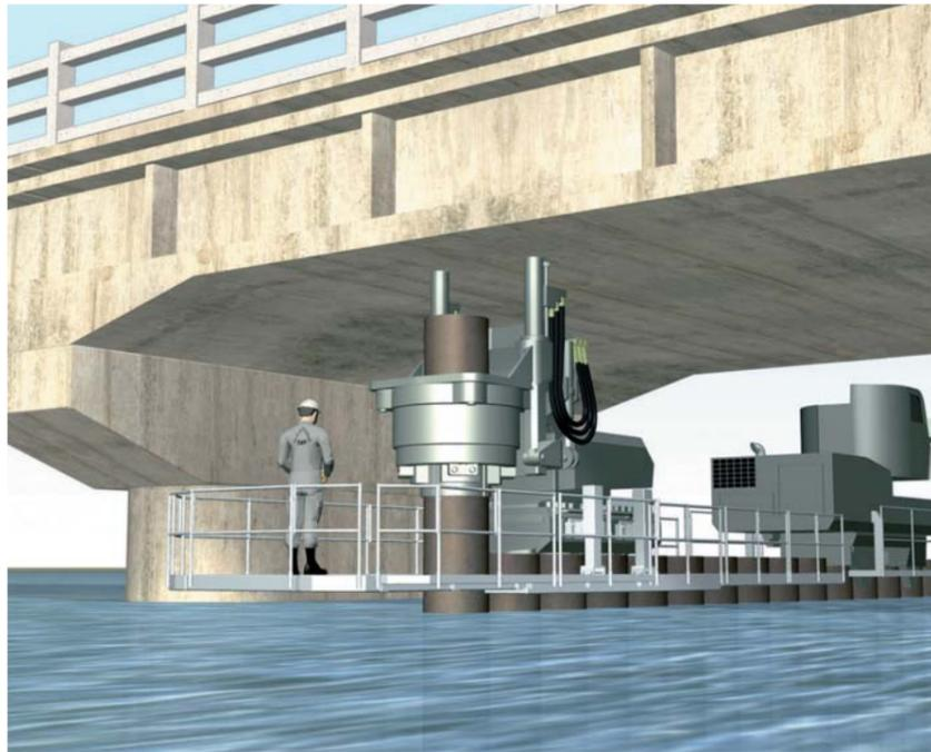
Construction work can be carried out at beneath overhead obstruction, because Gyro Piler is compact and gripping position of pile being pressed-in is close to the pile top of competed piles. Especially in case of severe height restriction, Gyro Clear Piler, a specially designed Gyro Piler with short height, should be selected.
