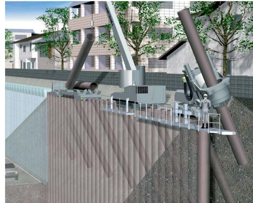
Gyro Piler has a lateral tilting function. It enables to install batter piles and anchor piles. Gyro Piler can construct high modulus retaining walls.
