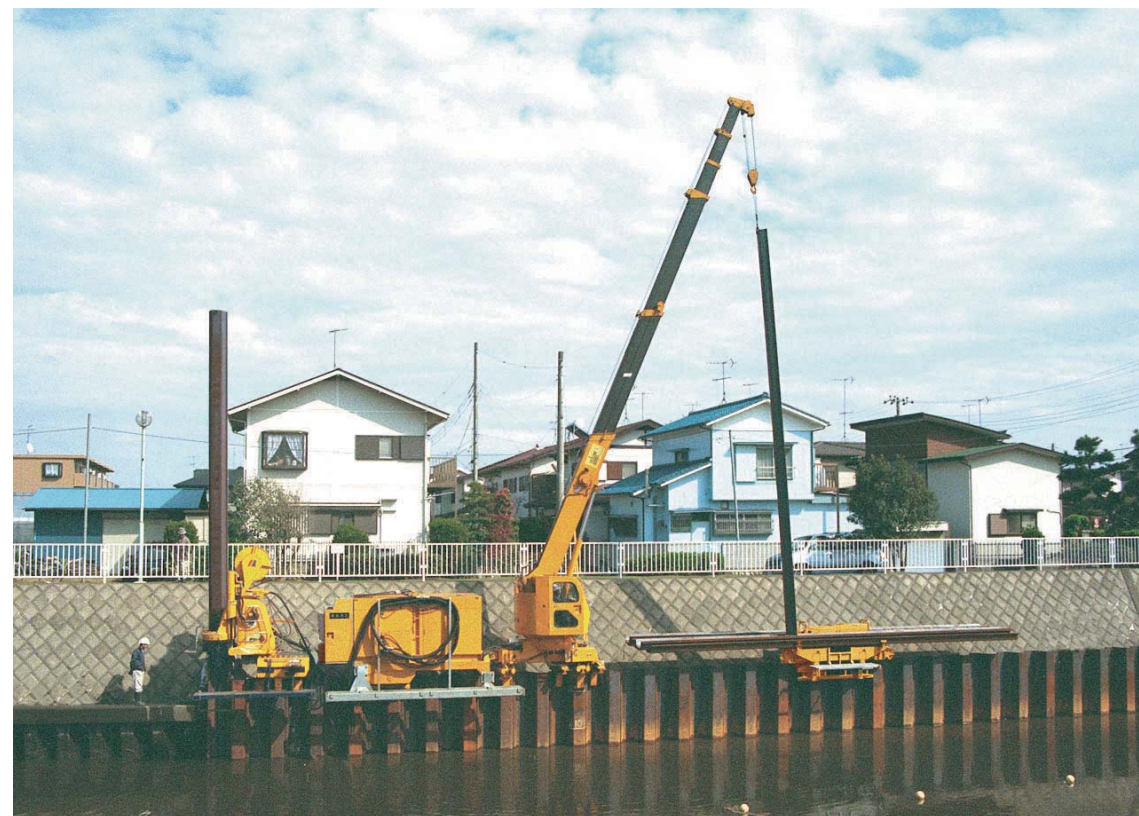
Flood Control Work in a residential area using the Non-Staging Method
